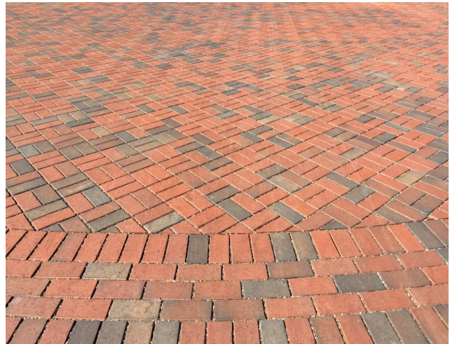
Photo 2 Permeable Clay Pavement
