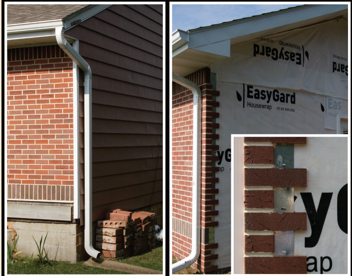
Insulation and thin brick can be placed over existing siding.
